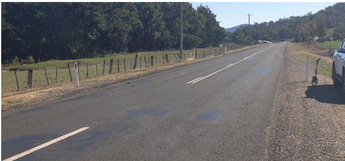
Image 7 – North bound on Nundle Road towards crest
