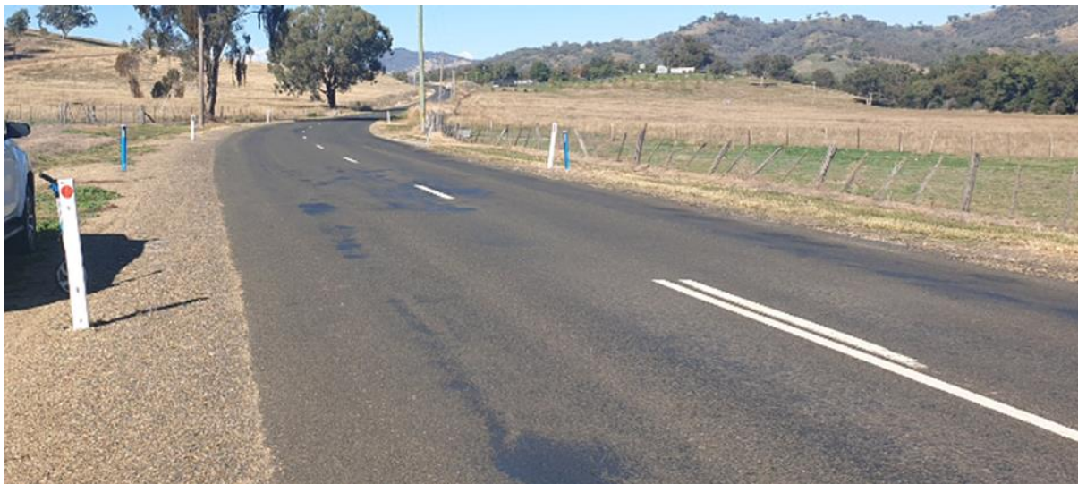
Image 8 – Southbound on Nundle Road away from crest
