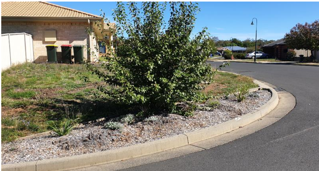
Image 10 – Bush restricting sight distance
